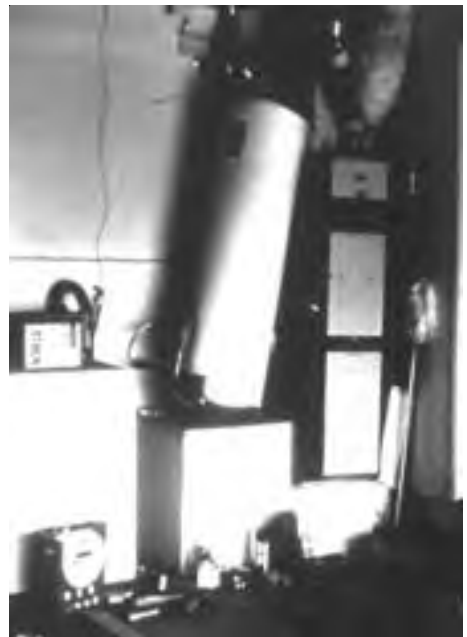
Figure 11 - This unstrapped water heater tipped over during the 1984 Morgan Hill Earthquake. Fortunately gas and water lines were not ruptured.
