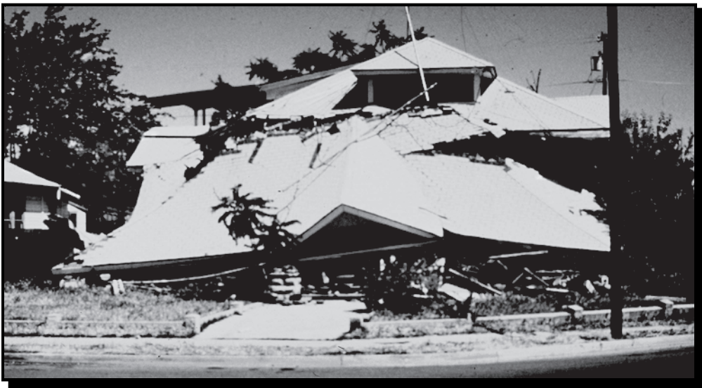
Additional damage from aftershocks
